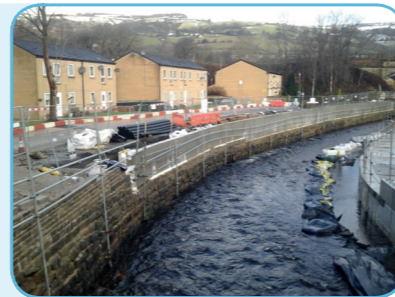
Installing permanent defences along Cragg Brook, December 2017
