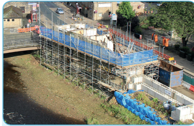
Demolition work along Burnley Road, Autumn 2017
