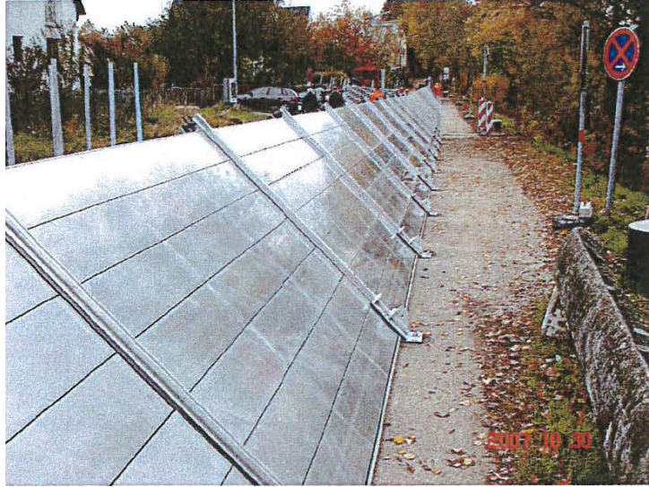
Figure 2: Typical installation of a K-Barrier System
