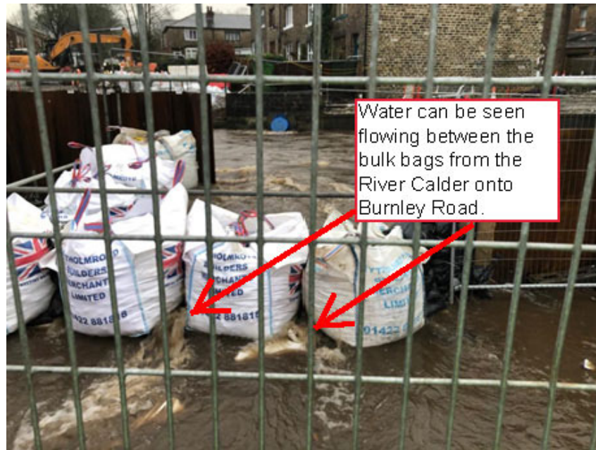
Figure 10: Image showing L-type arrangement of bulk bags
