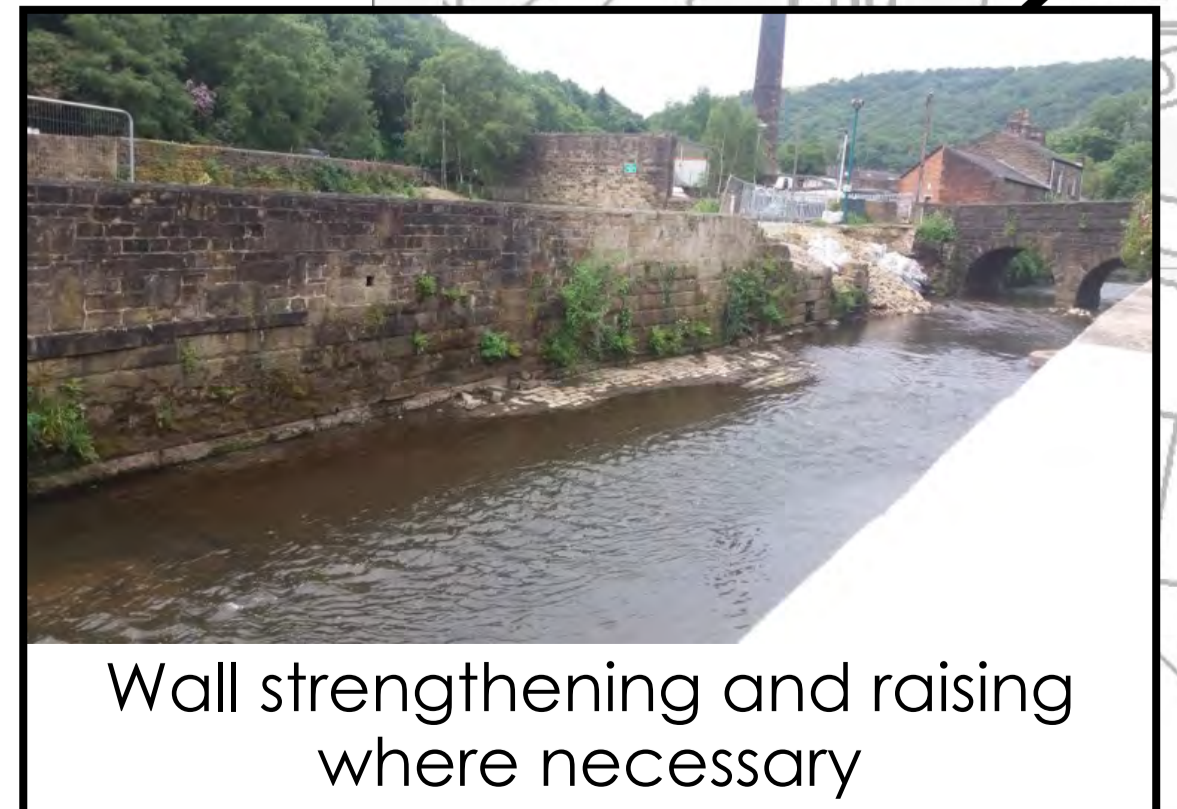
Increase wall heights along Stubbings Lane in keeping with the visual characteristics of the town
