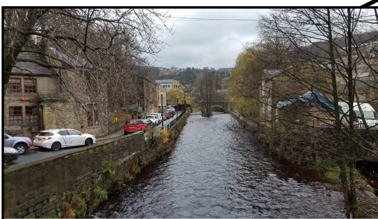
New Road Bridge - looking north
