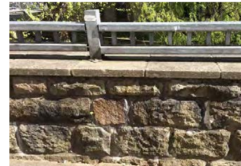
Existing stone wall in Hebden Bridge with coping stone
