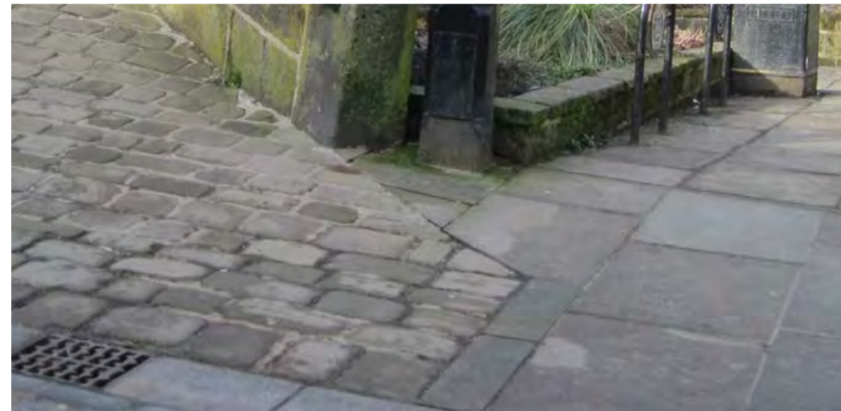
Paving detail on Bridge Gate
