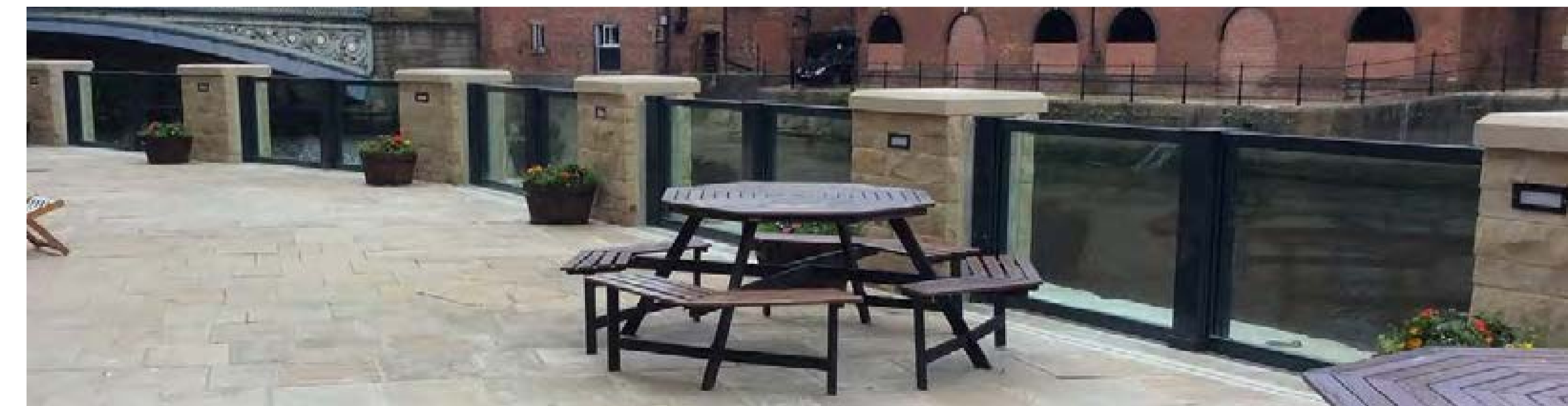
Stone clad flood wall with inserts of full height glass © EA
