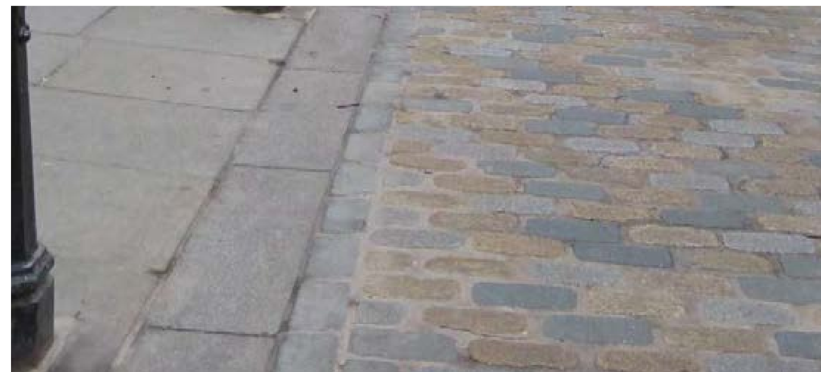
Paving detail on Bridge Gate
