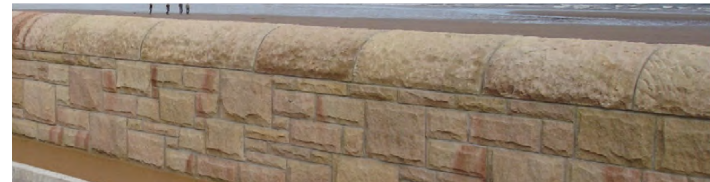
Carnoustie Wall - random coursed pitched face wall in sandstone © Tradstocks 'Overwood' - Tradstocks LTD
