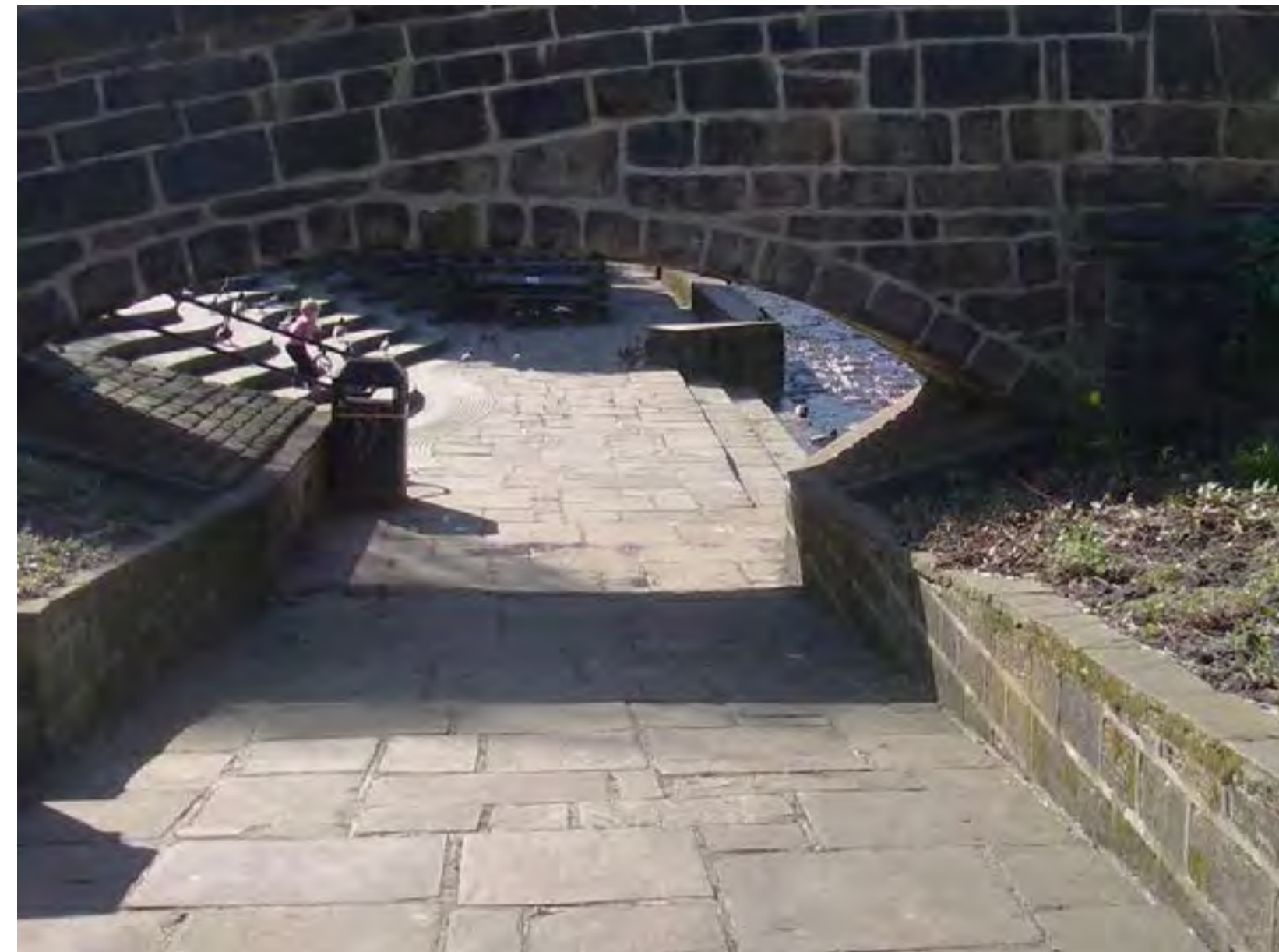
View of ramp near the Packhorse Bridge
