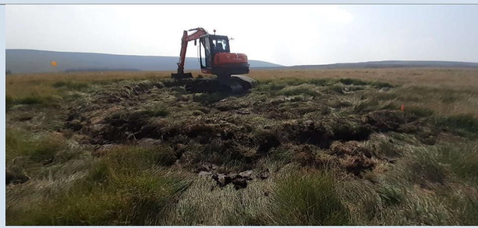
Installation of peat bunds above Hebden Bridge (© Moors for the Future)
