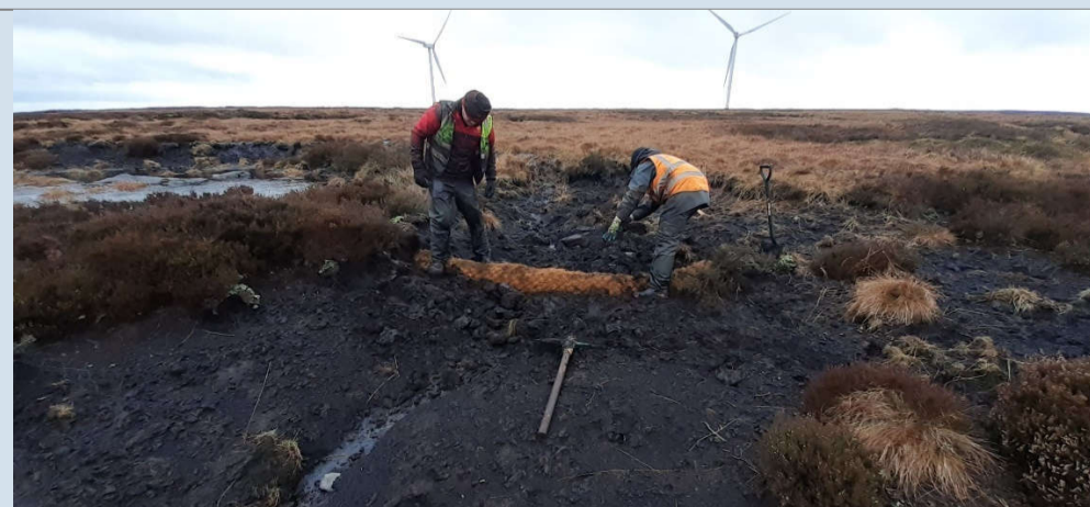
Installing gully blocks above Mytholmroyd (© Moors for the Future)
