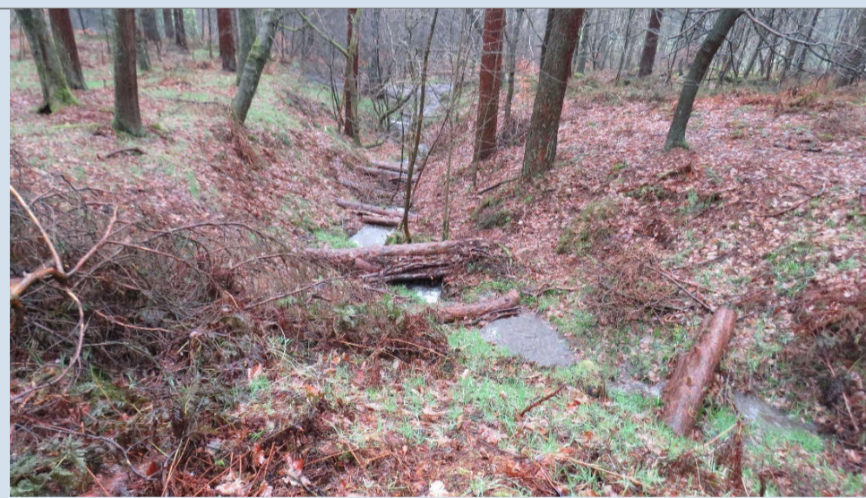
Leaky Dam implemented in Calderdale (© Stuart Bradshaw)
