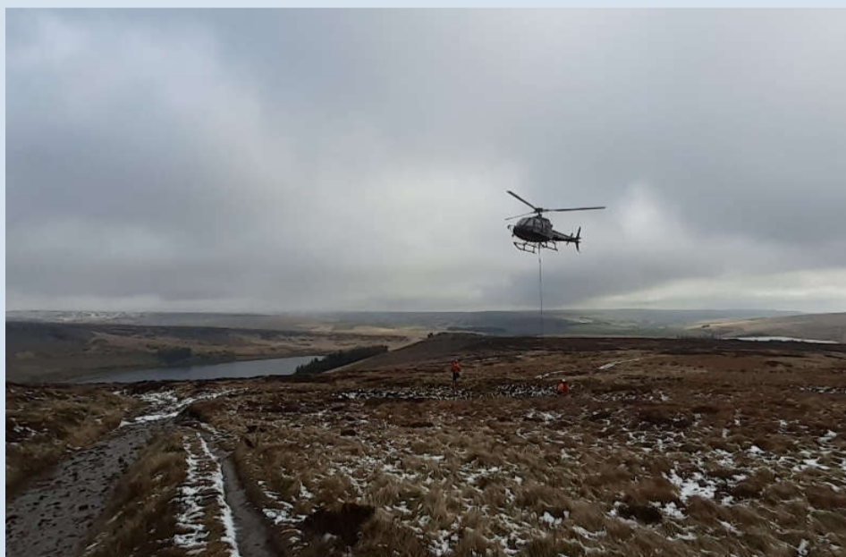
Installation of stone dams (© Moors for the Future)
