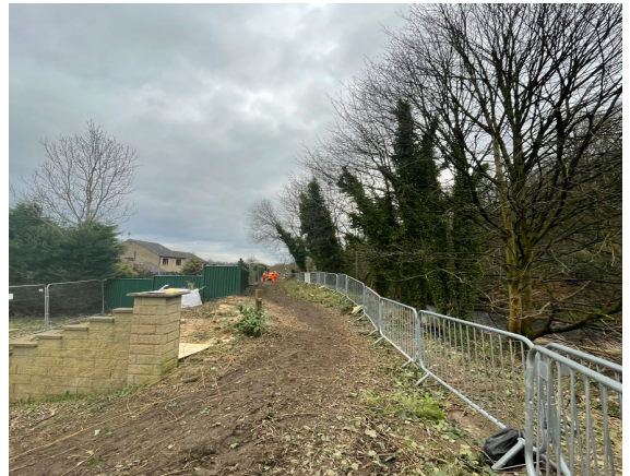
Photograph: after de-vegetation work
