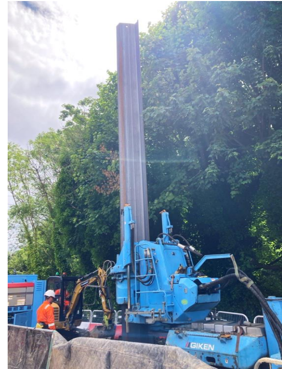
Hydraulic press used to install sheet piles.
