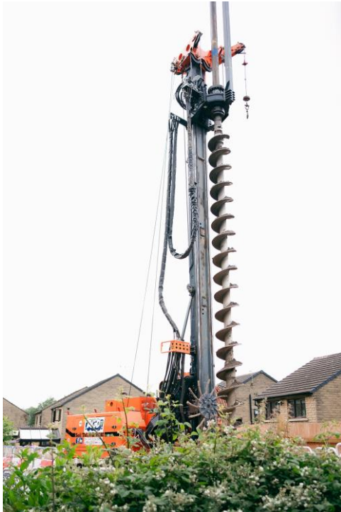
Pre-auger used to prepare ground for piles.
