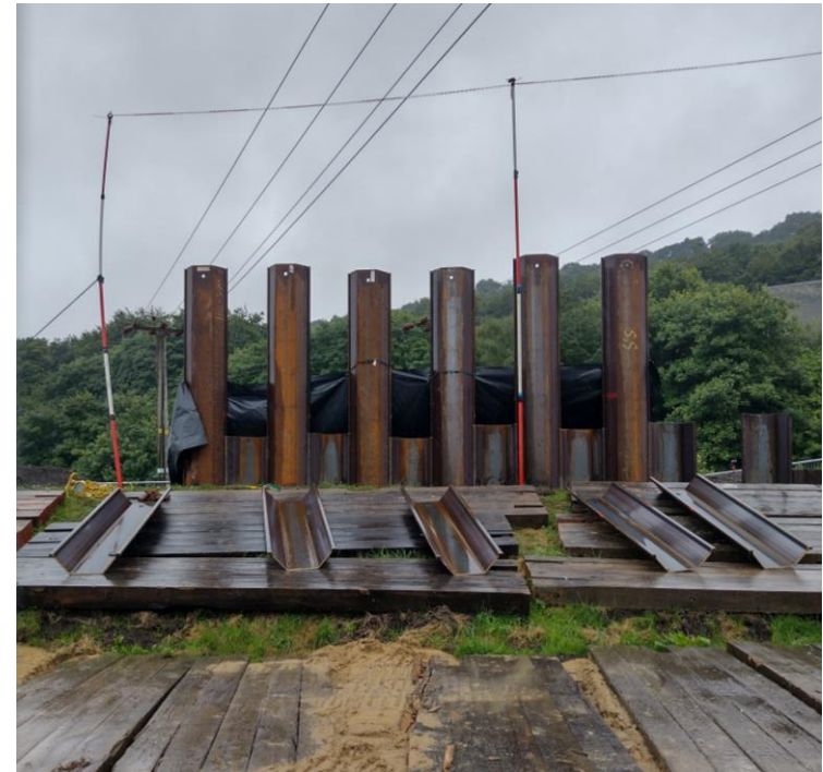
Piles being installed at rugby club embankment.
