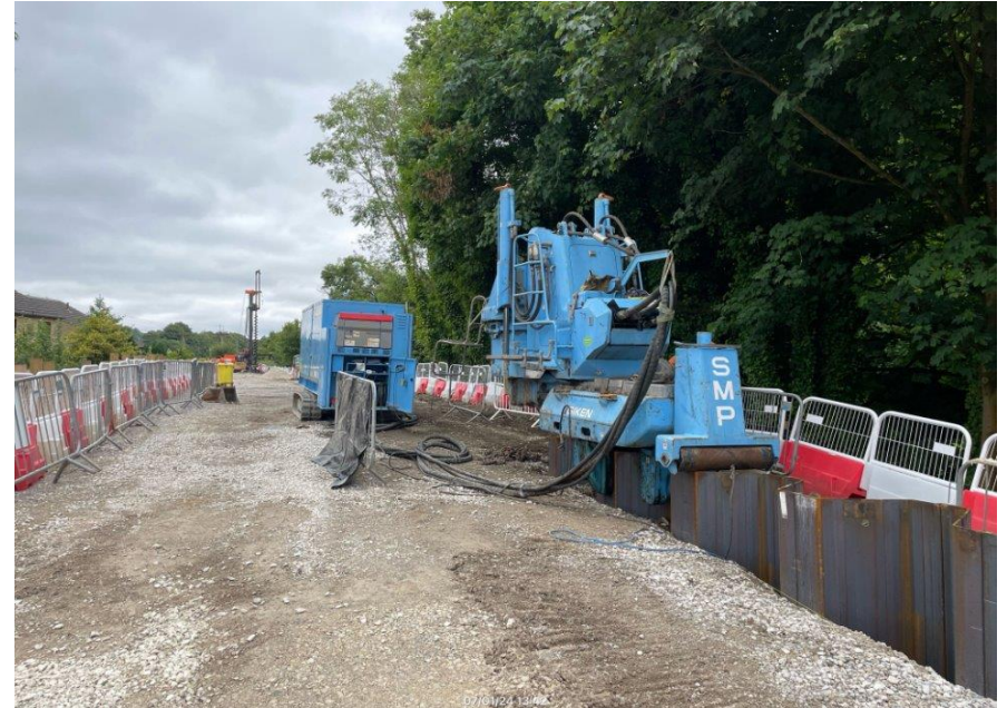
Hydraulic press installing piles.
