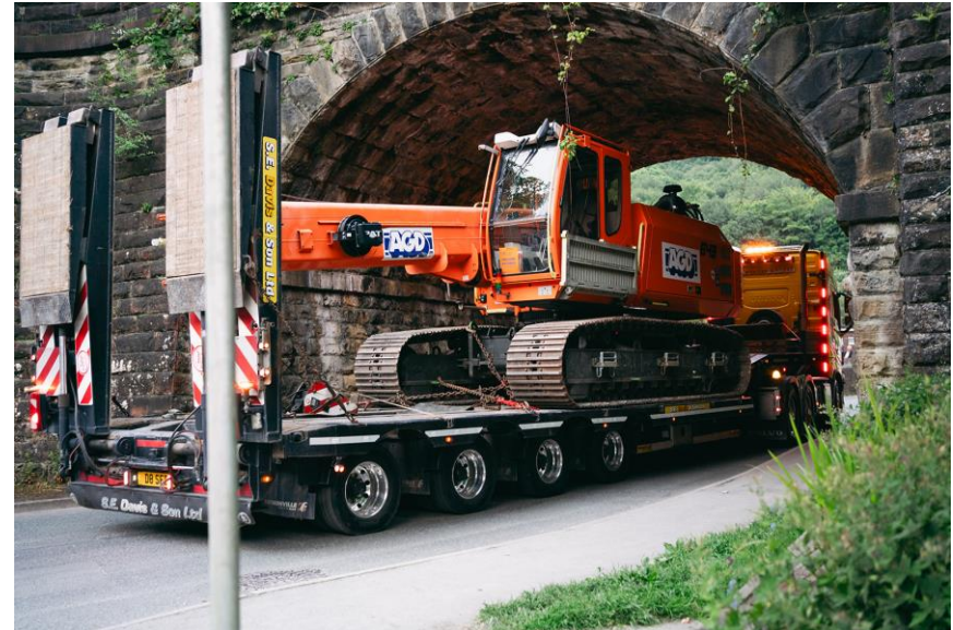
Crane being delivered to Copley.
