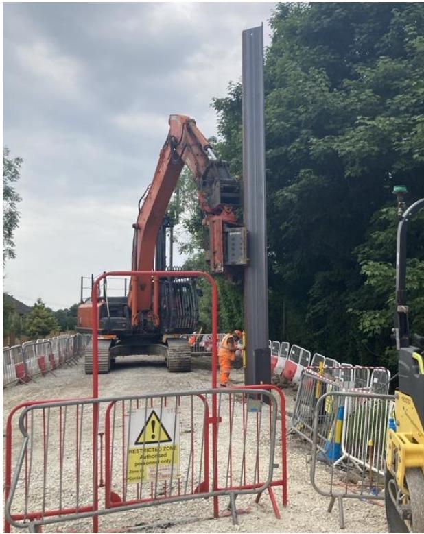
Movax unit installing starter piles.
