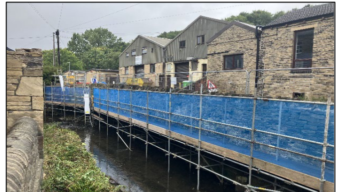
Scaffolding for wall repair access
