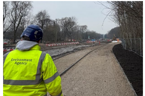
Ongoing construction of new footway/cycle
