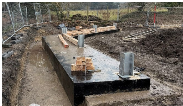
Weir base construction
