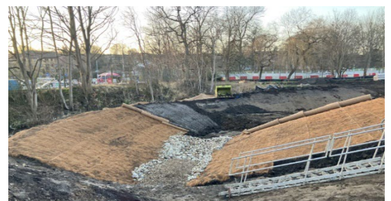
Clifton Beck Channel realignment
