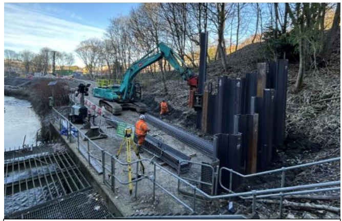
Sheet pile installation
