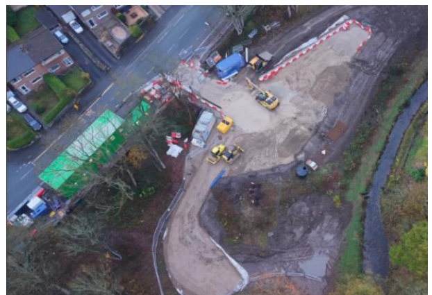
Site cabins and temporary site access
