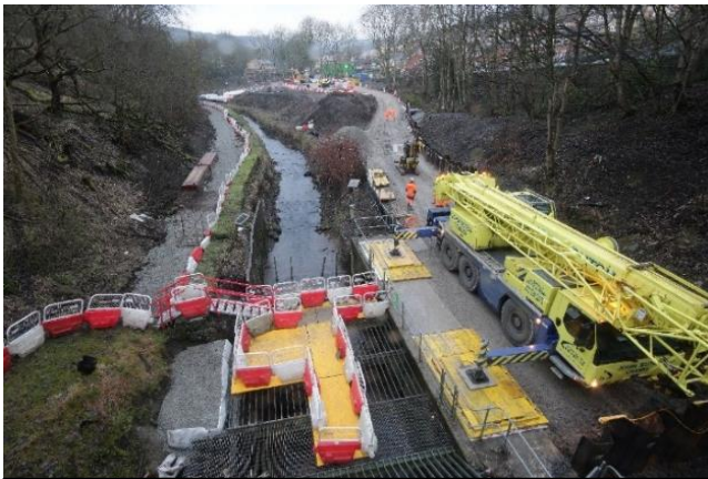
Overview of the site
