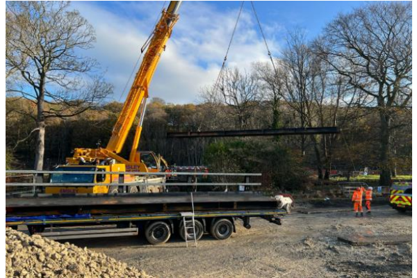
Temporary Bridge being removed
